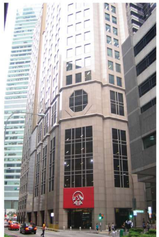
AIA Tower Singapore
